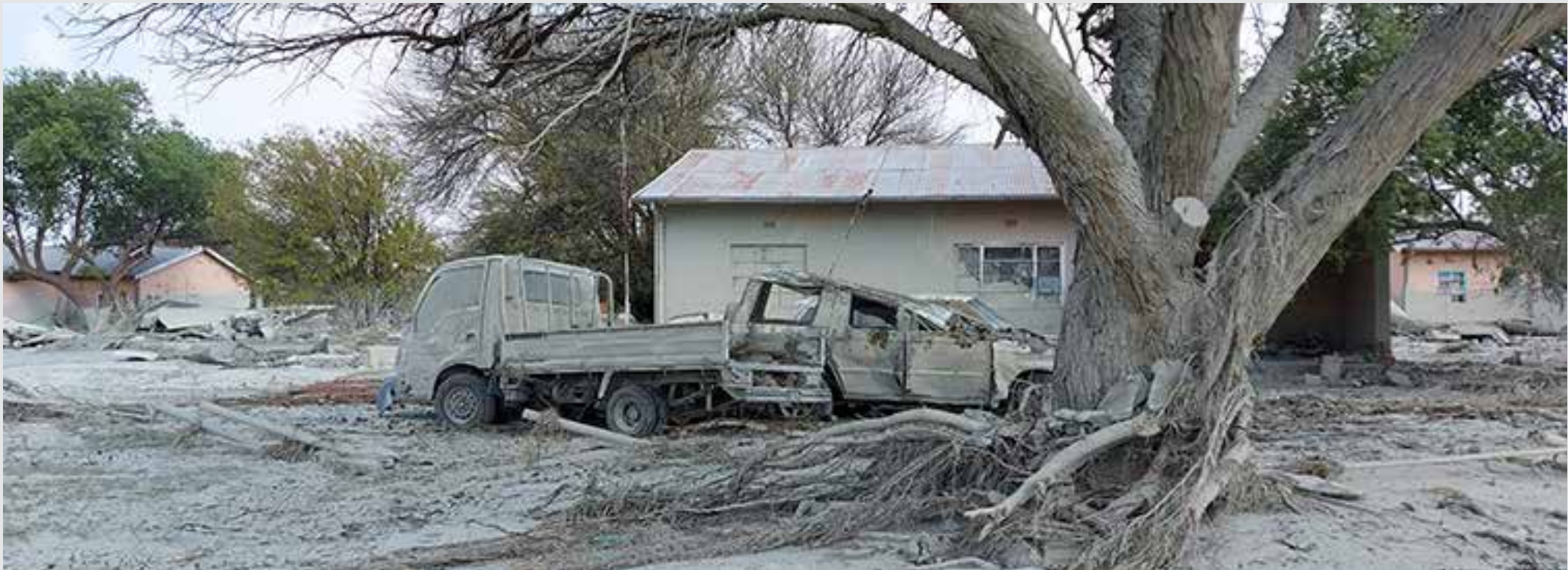
The aftermath of the Jagersfontein tailings dam collapse on 11 September 2022, which released millions of cubic metres of mining slurry, claimed two lives, damaged approximately 200 homes, and contaminated around 1 600 hectares of agricultural land. Pictures: Dr Anita Venter
