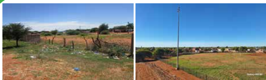
The Upgrading of the Sports Field in Dibeng
