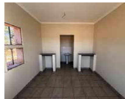
Internal Refurbished clubhouse
