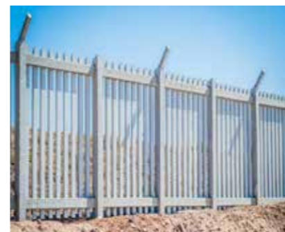
Replaced perimeter fence
