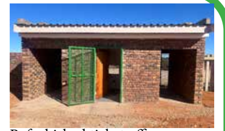
Refurbished ticket office
