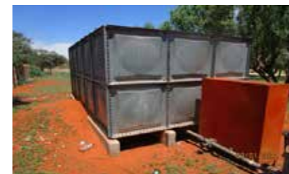
Old tank/ reservoir
