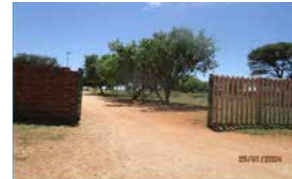
No gate on site
